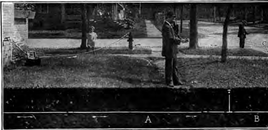
FIG. 284. — Manner of Using Wireless Pipe Locator.
